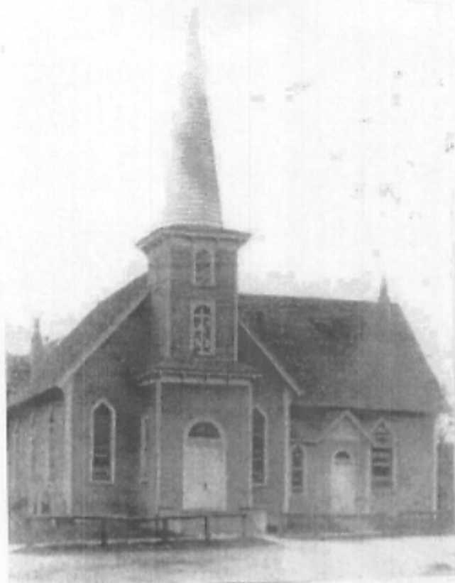
Frankford United Methodist Church Main Street
