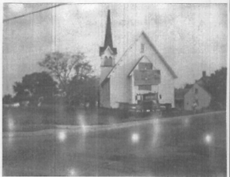
Frankford Presbyterian Church being Moved from Reed Street to Present Location on Main Street
