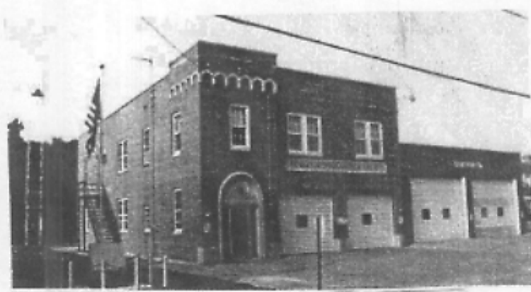
Fire Hall with Additional Bays
