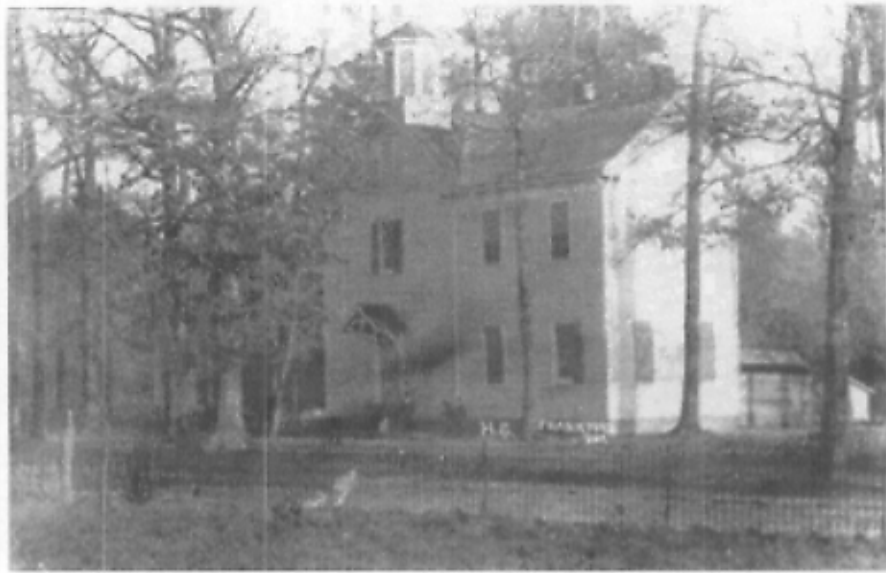
Old Frankford School Thatcher Street
