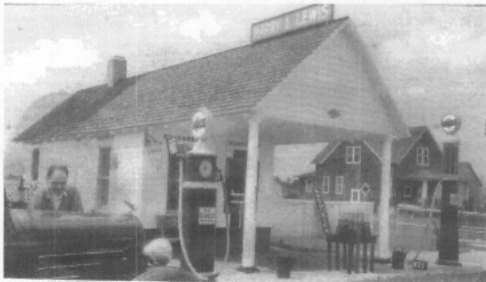
Harry & Wilmer Lewis' Store & Service Station DuPont Highway
