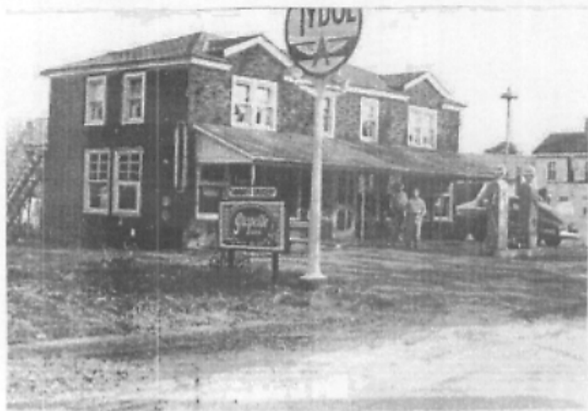
Carson Thomas' Store Clayton Avenue
