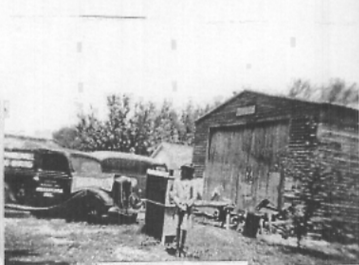
Russ Parsons Garage Clayton Avenue
