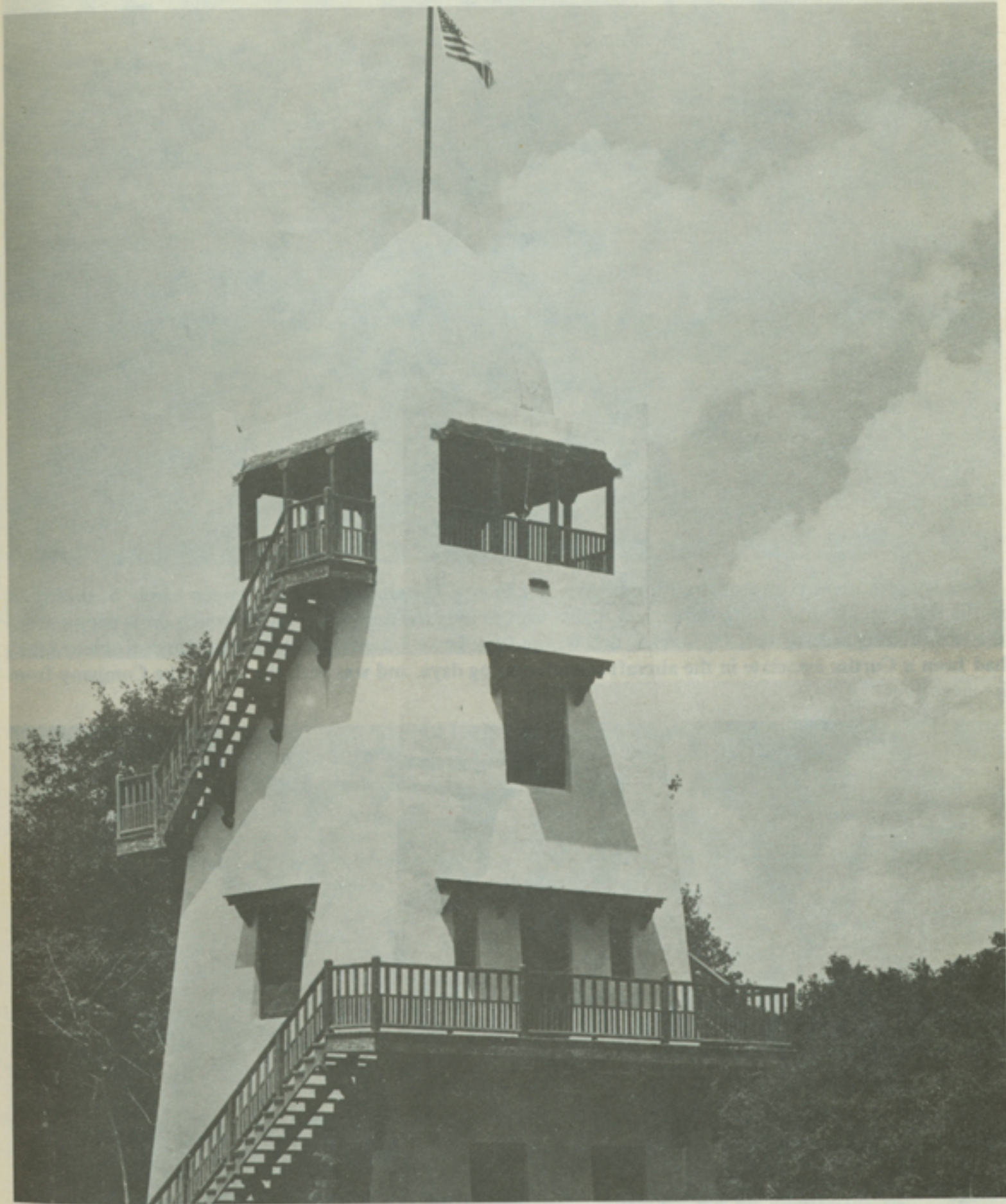
Observation Tower, designed by Mr. Muller, which stood north of Cook's Hammock (Opa-locka Park) and west of the Florida Aviation Camp's landing field. From it one could command a view northward and westward across the golf course and eastward across the city. It is my recollection that it was still standing when we first revisited the city of Opa-locka in January of 1937. On our return in 1940 it was gone, probably demolished, along with the park and golf course, to make way for expansion of the Naval base.
